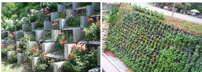
Figure 8. Examples of compound views (Right) the use of concrete blocks (from: khakemosalah.ir ), (Left) the use of plastic baskets (from: www.miracell-ccs.com )
