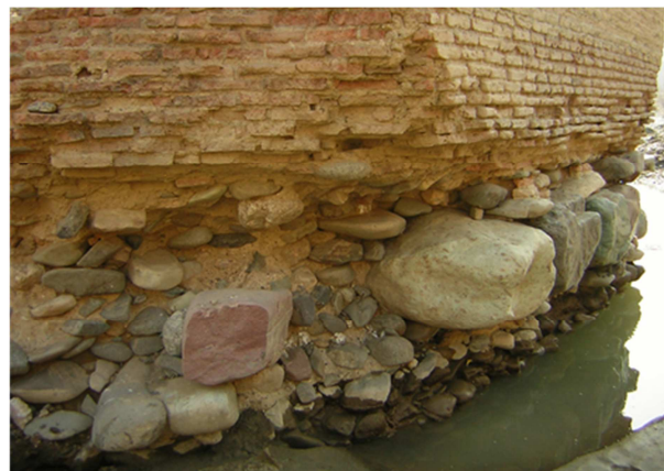
Figure 23. Foundation of the medial vault, before restoration 2006.
